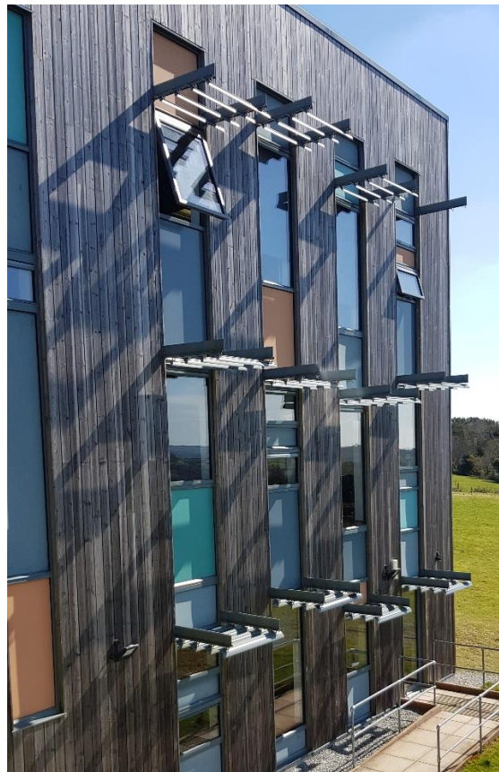
Figure 5.1: Brise Soleil Shaders on a South Facing Office Building
