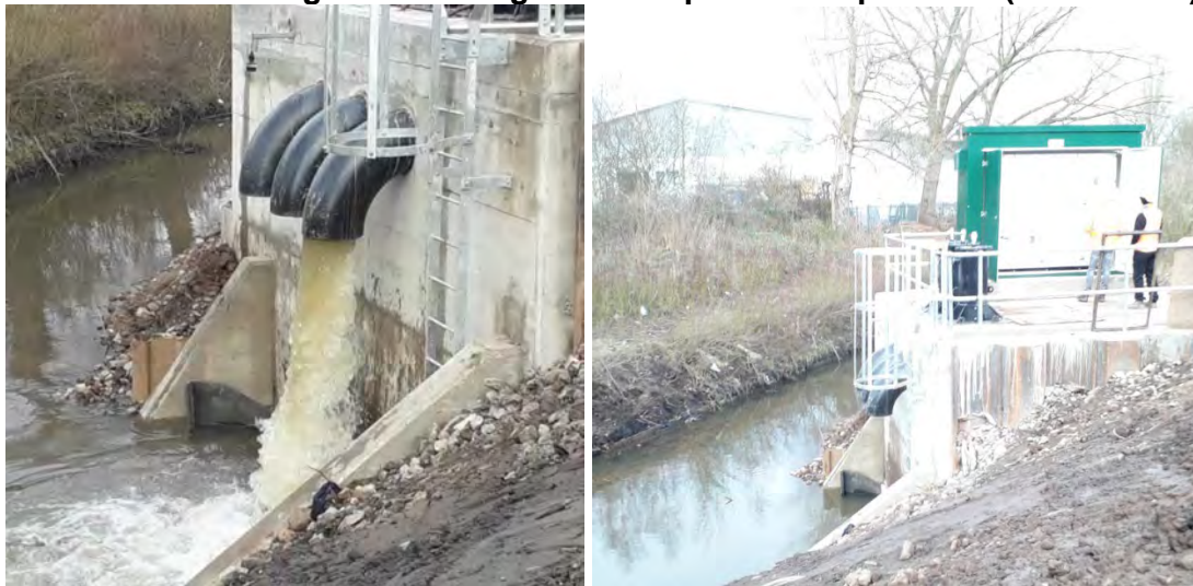
Figure 185: Images of Completed Pump Station (March 2021)
