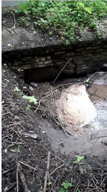
Figure 86: Image of Culvert on 26 May 2021.
