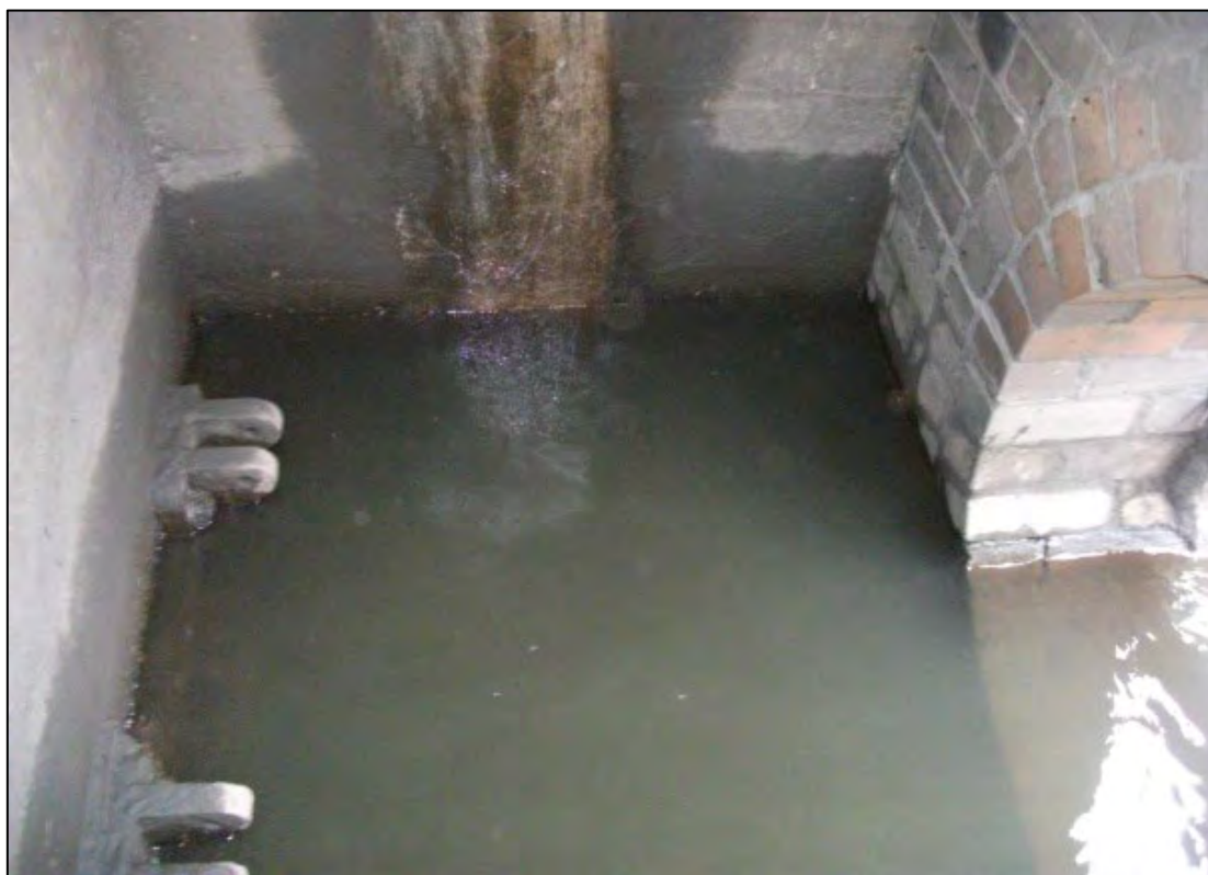
Figure 182: Image of Inside Outfall Chamber to Dallam Brook
