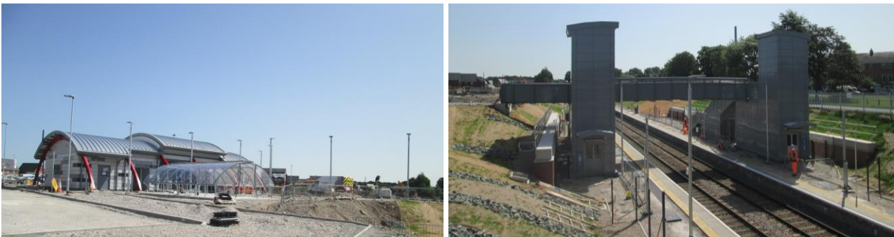
Figure 10.3 -Warrington West Station Construction Work
