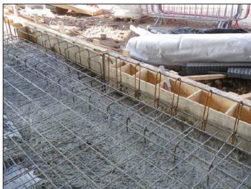
Concreting at GL A 16-19
