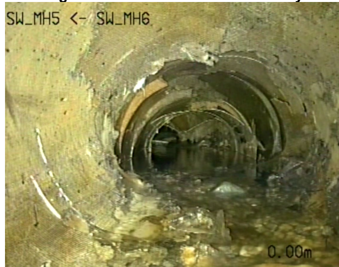
Figure 15: Extract from CCTV Survey
