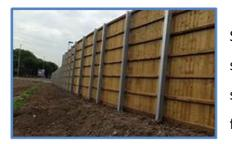
Suitable for new residential to mitigate against existing noise sources including busy road or industrial. Need to consider the scale and type of barrier and future maintenance and liabilities for repairs.
