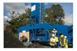
Remediation methodologies include 'biostimulation', which encourages the natural attenuation of soil contaminants and 'bioaugmentation', which relies on the introduction of micro-organisms to promote and enhance degradation of contamination.
